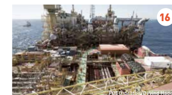
PEREGRINO FPSO, STATOIL O&M contract
