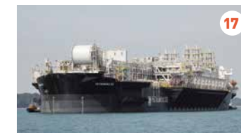
P-63 FPSO, PETROBRAS EPC, O&M contract
