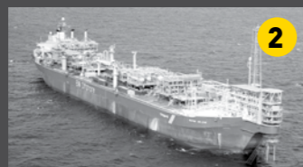
BERGE HELENE FPSO, PETRONAS
