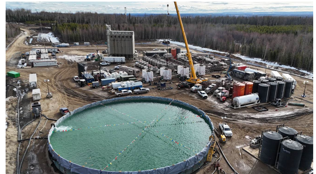
Completion Operations on Kakwa North
