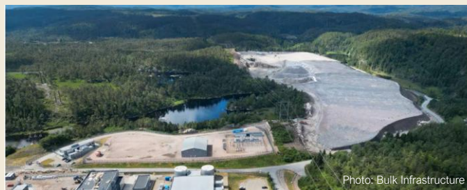
Project: N01 Campus Støleheia HV EPCM Customer: N01 Utilities AS Period: 2026 – 2029
