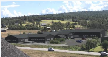
High-volume robotised manufacturing (Røros)
