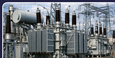
Goodtech awarded contract to upgrade Skistua transformer station in Narvik
