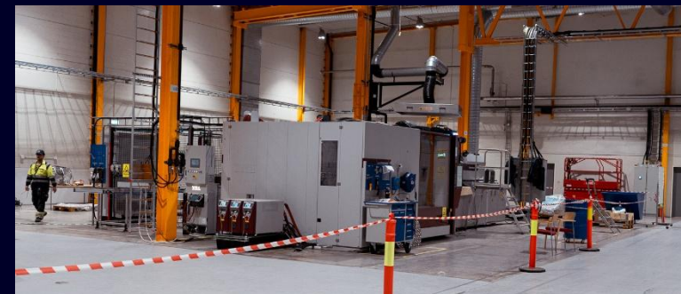
New pressurized alkaline production line progressing according to plan
