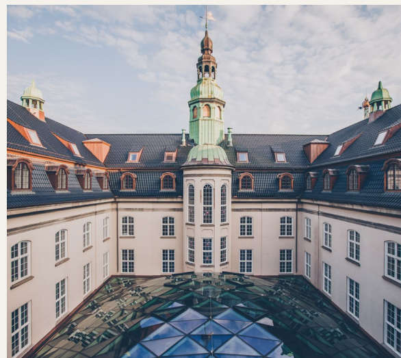
Photo: Villa Copenhagen
