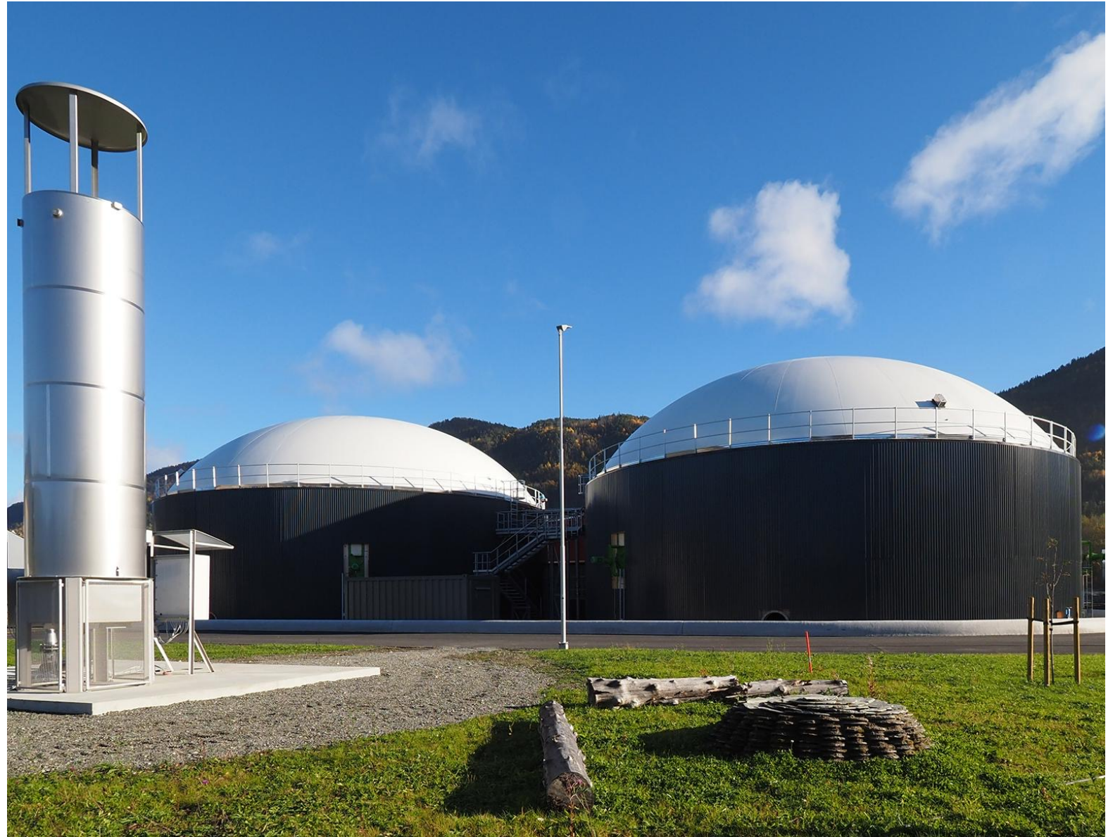
Voss Biogas Plant | Photo: LINK Arkitektur / Bjørn Feltens
