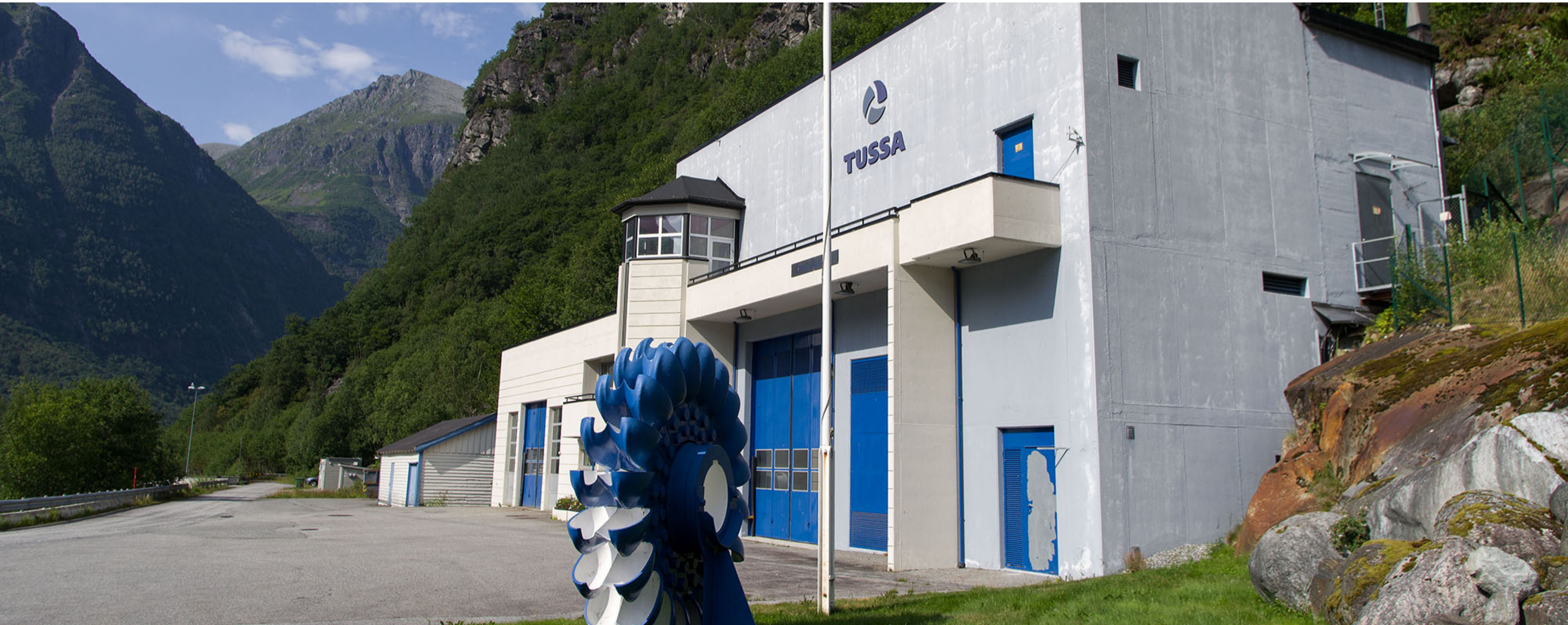
Tussa II power plant, Norway | Photo: Knut Hustad
