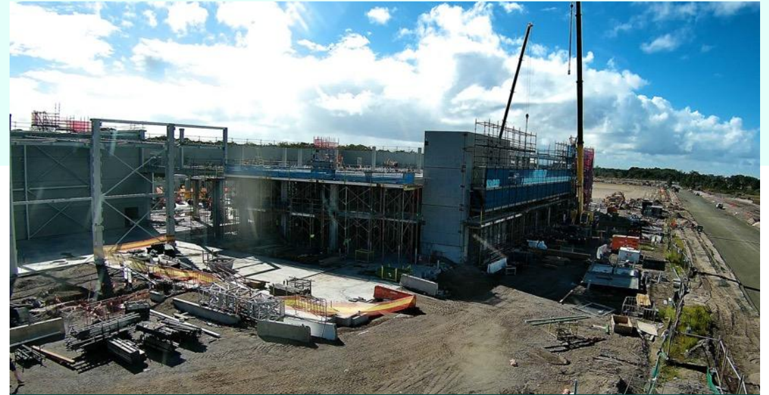
Newcastle, Australia Virginia, USA
