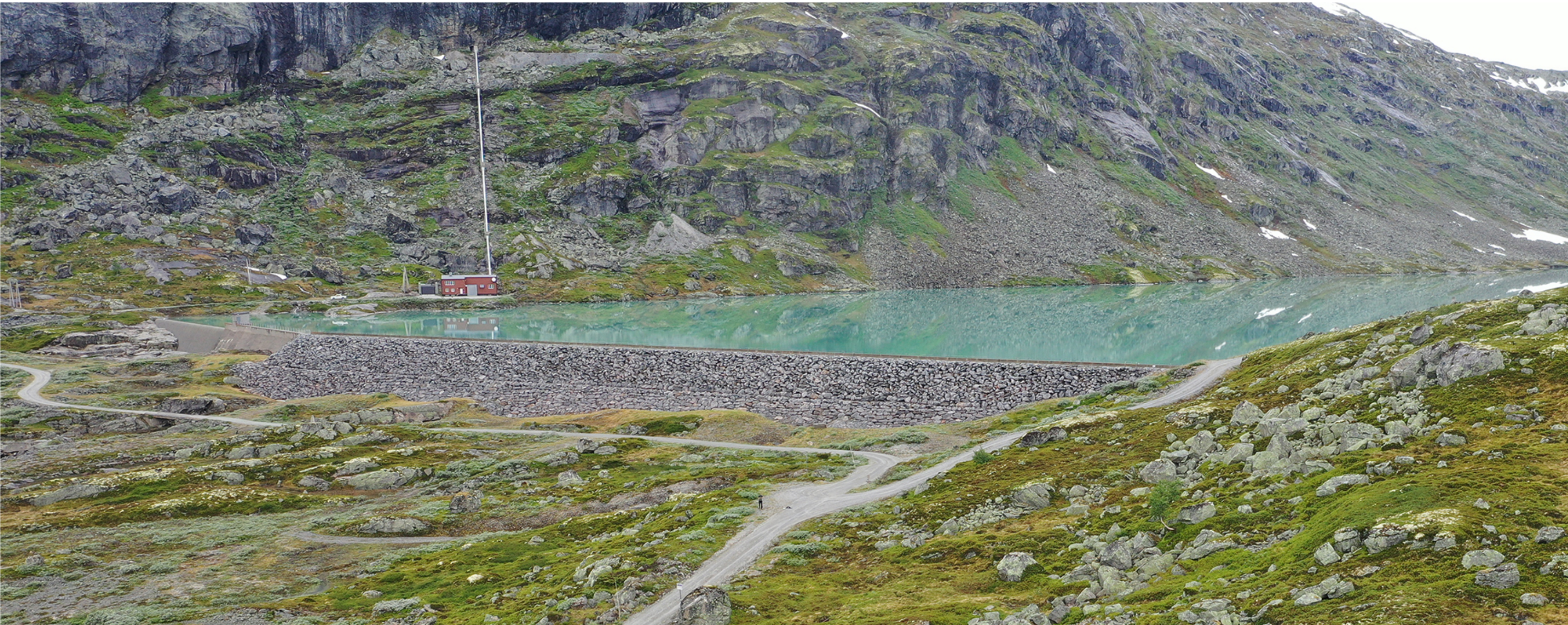
Illvatn pumped storage plant, Norway
