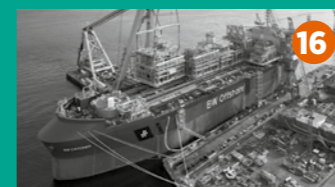
16 BW CATCHER, PREMIER OIL (Under construction)
