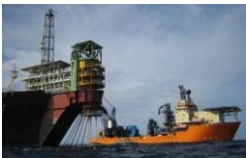
External Turret Production (ETP) for FPSO
